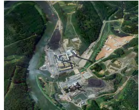
Aerial view of the Black Warrior Basin Gorgas Power Plant site. (Image courtesy of Google Earth, U.S. Geological Survey, and USDA Farm Service Agency)
