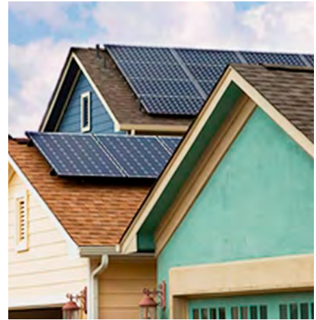
Rooftop solar panels increase energy efficiency on homes in Austin, TX. (Image courtesy of Donald Geiling)
