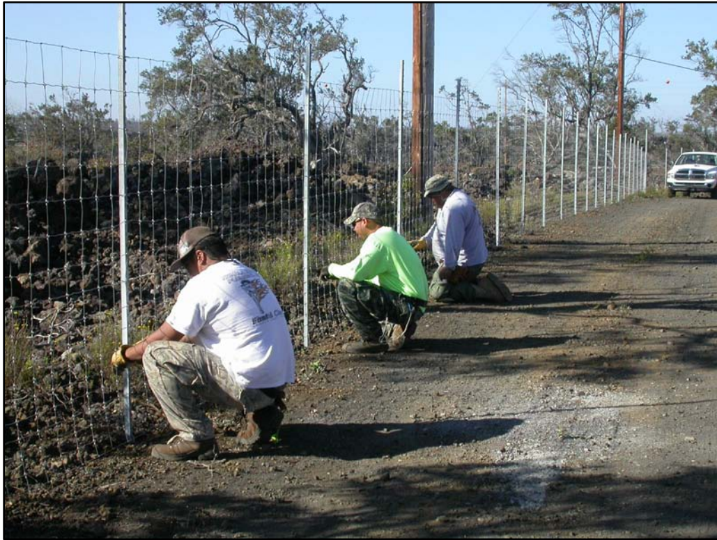
Figure 4.0-1. Fence Crew clipping wire mesh to T-posts.
