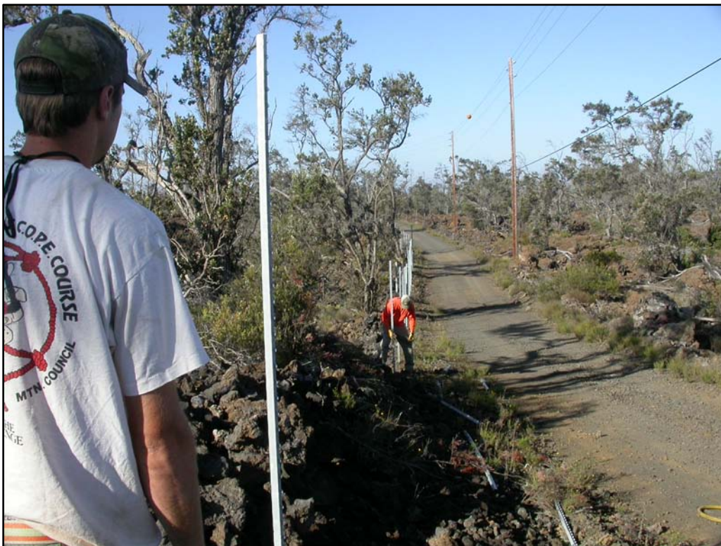
Figure 4.2-2. Fence Crew aligning and setting posts.
