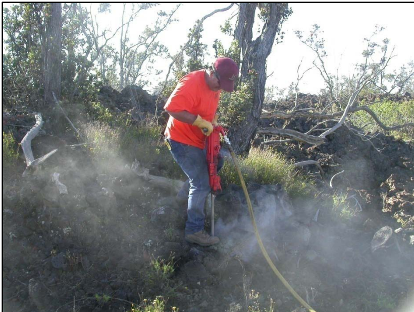
Figure 4.2-1. Drilling post-holes in rock.
