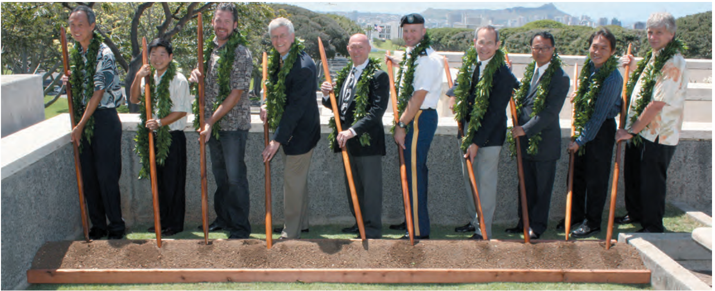
Leaders from the U.S. Army Corps of Engineers joined officials from the Veterans Administration, the American Battle Monuments Commission and others on May 9 to break ground and bless the new Vietnam Pavilions Project at the National Memorial Cemetery of the Pacific at Punchbowl. From left to right: Honolulu District Chief, Military Branch, Andrew Kohashi; Honolulu District Project Manager Jason Tanaka; Contractor Mike Gangloff; ABMC Chief of Staff Michael Conley; Director, National Memorial Cemetery of the Pacific Gene Castagnetti; Honolulu District Commander Lt. Col. Douglas B. Guttormsen; ABMC Director, U.S. Memorials, Thomas Sole; President Fung Associates Louis Fung (architect); Contractor Paul Wong and State of Hawaii Department of Land and Natural Resources Deputy Director William Tam. Photo by Joseph Bonfiglio
