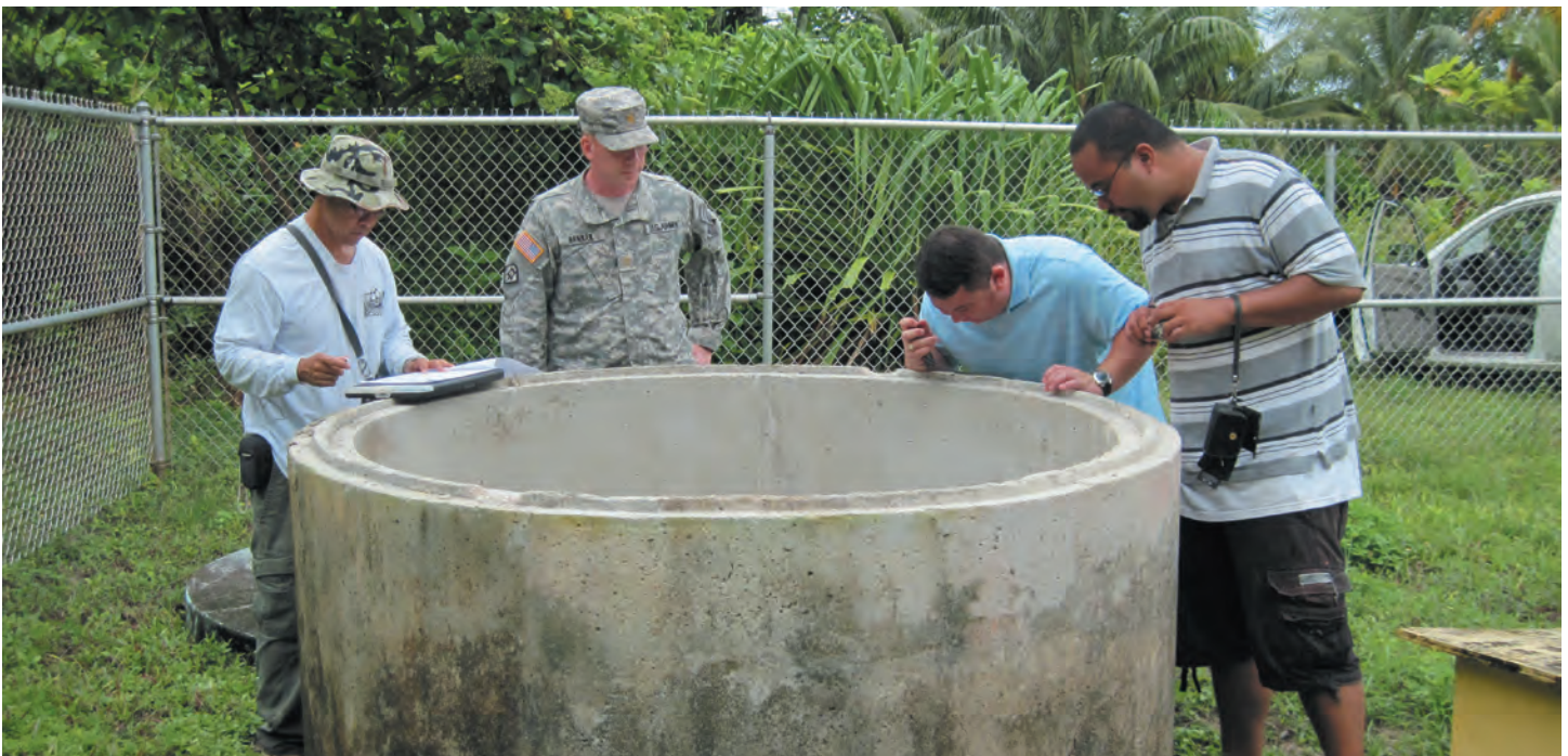
(Left to right) Mechanical Engineer Jon Hosaka records observations as 565th Engineer Detachment Commander Maj. William Hannan and Civil Engineer David Nishimura inspect a water well along with the Majuro Water and Sewer Company operations manager during the 565th's week-long infrastructure survey mission in August. Photo by Alan Avery
