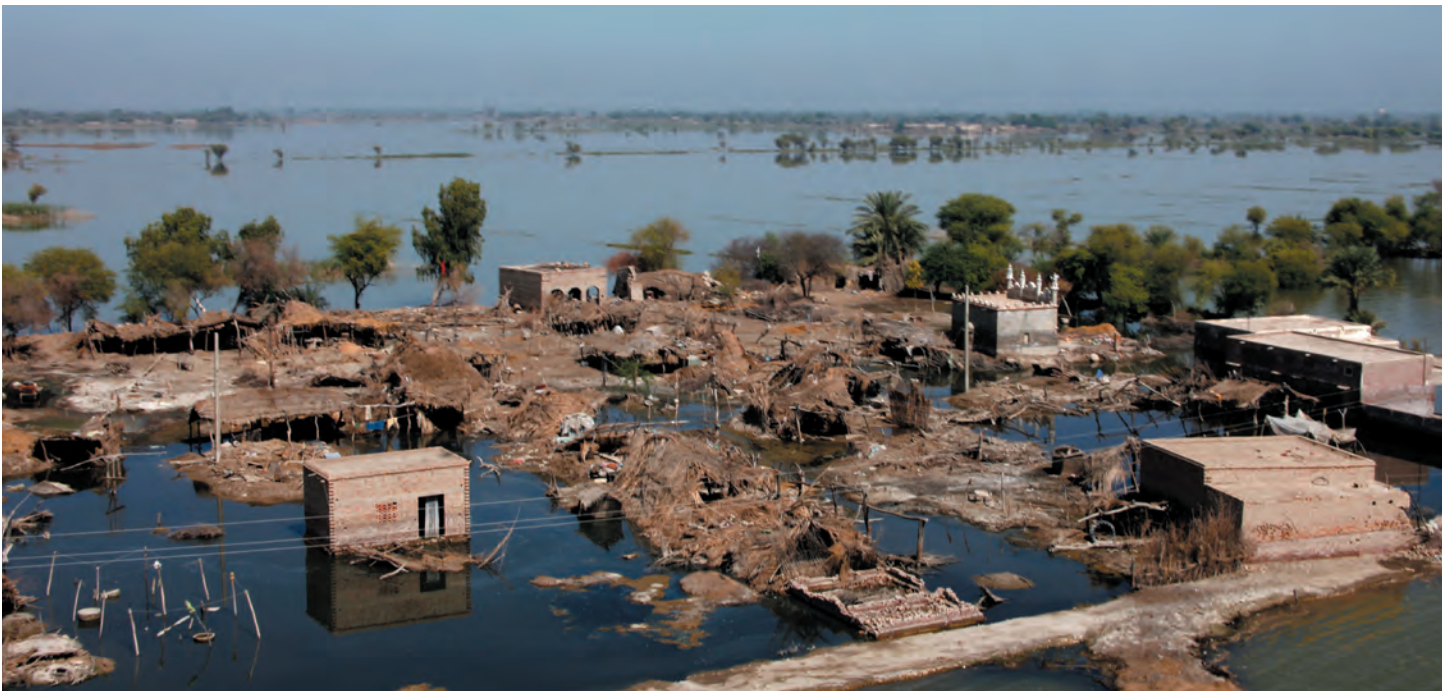
Damages in the flood-affected areas in the Sindh province after a monsoon season in Pakistan. U.S. Marines with the Marine Medium Helicopter Squadron 165 Reinforced, 15th Marine Expeditionary Unit and the Marine Medium Tilt Rotor Squadron 266 Reinforced, 26th Marine Expeditionary Unit assisted the Pakistan Army with humanitarian assistance operations. Courtesy Photo
