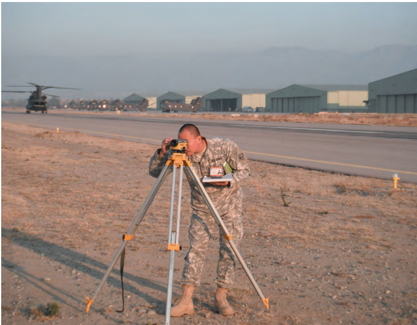
Maj. Evan Ting verifies landscape survey readings on the Chaklala Air Base flightline to assist in compiling a layout for a 300-personnel base camp near the Pakistani capital of Islamabad. Courtesy photo
