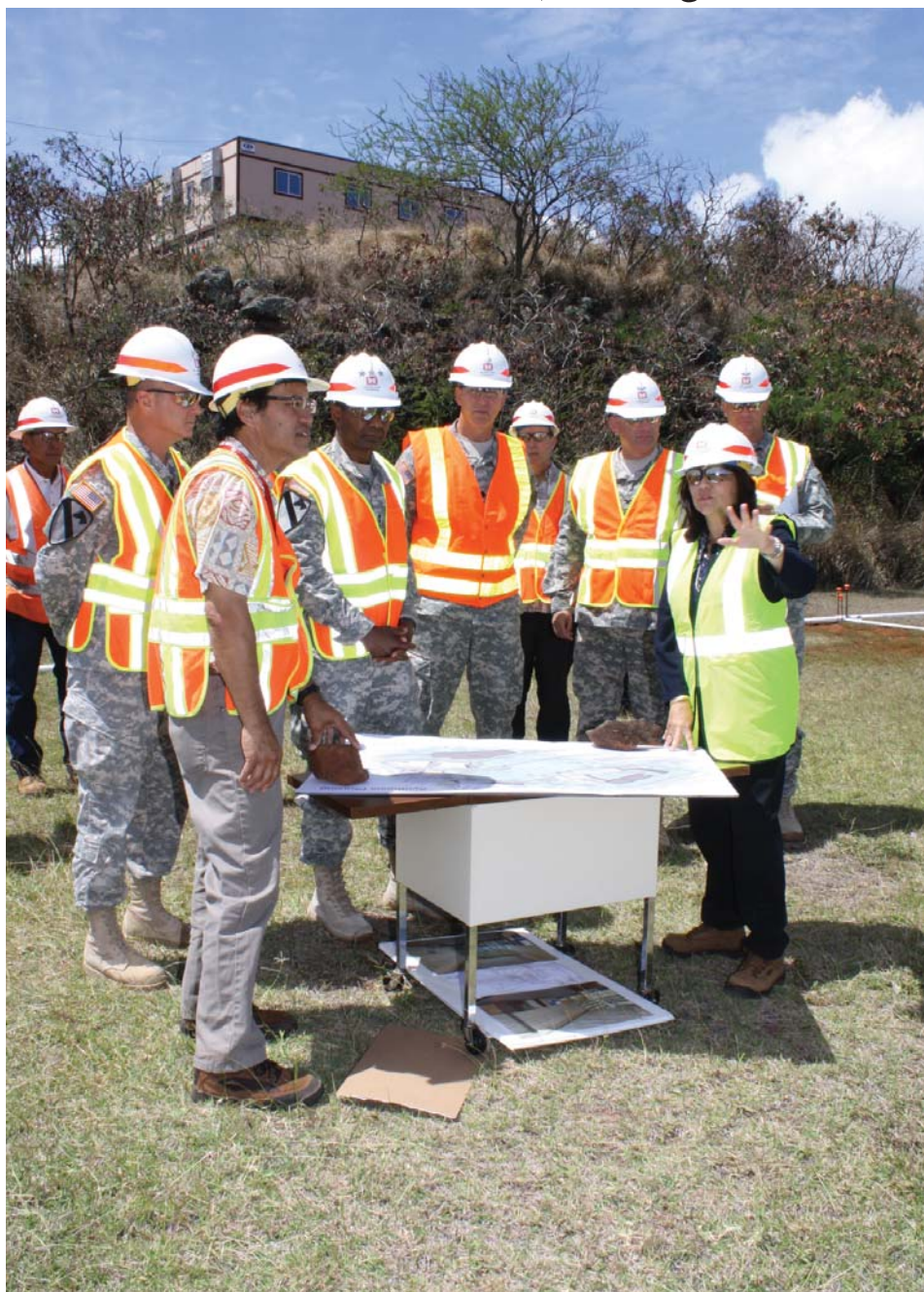
Commanding General U.S. Army Corps of Engineers Lt. Gen. Thomas P. Bostick (front row, third from left) listens as Command and Control Facility (C2F) Program Manager / Project Manager Lise Ditzel-Ma explains the project site layout of the future headquarters for U.S. Army Pacific during a visit July 23. Listening are (front row left to right) Maj. Gen. Kendall P. Cox, deputy commanding general U.S. Army Corps of Engineers (USACE), C2F Phase One Project Engineer Gerald Young, Lt. Gen. Bostick, Honolulu District Commander Lt. Col. Thomas D. Asbery, Honolulu District Fort Shafter Area Office Engineer Tim Phillips, Col. Robert Sinkler, strategic planner USACE, Ditzel-Ma and Col. Peter Andrysiak, executive officer, USACE. Photo by Dino W. Buchanan
