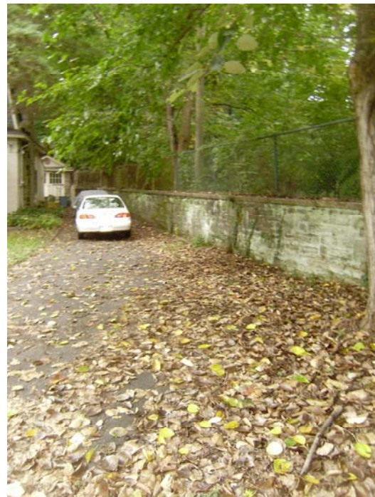
Figure 9: Wall adjacent to Tookany Creek overtopped in 2011.
