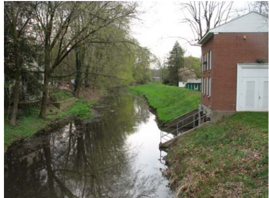
Figure 1: View looking upstream along Tookany Creek at Rice Mill Road. Pump Station is shown on the right.
