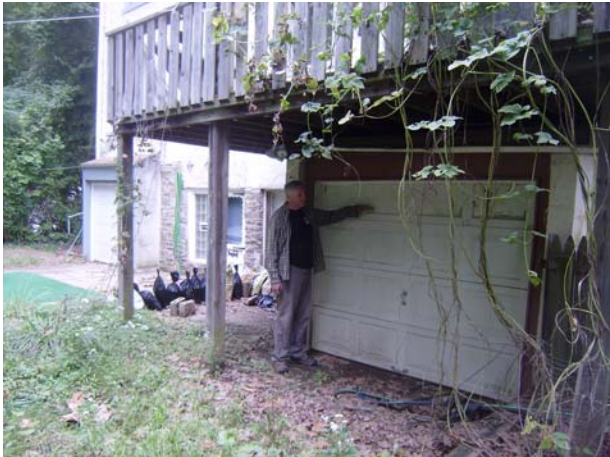
Figure 7: High water mark from the 2011 Events behind High School Road.
