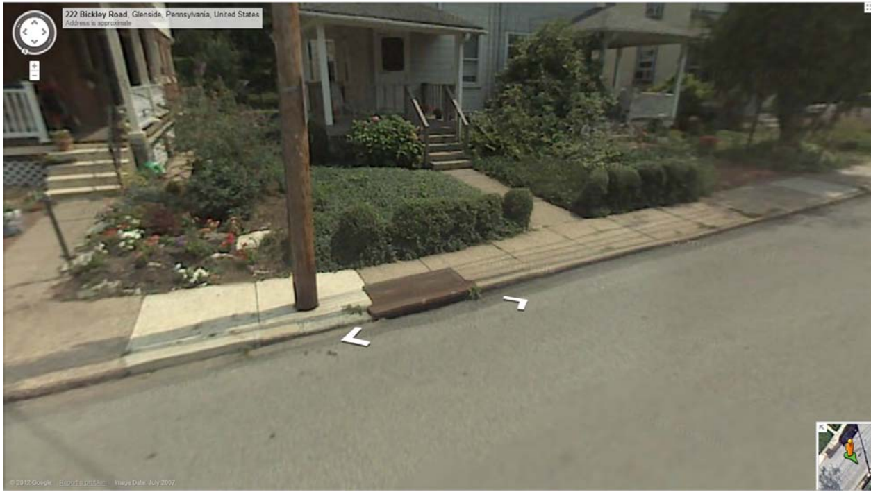
Figure 5: Single storm inlet along Bickley Road
