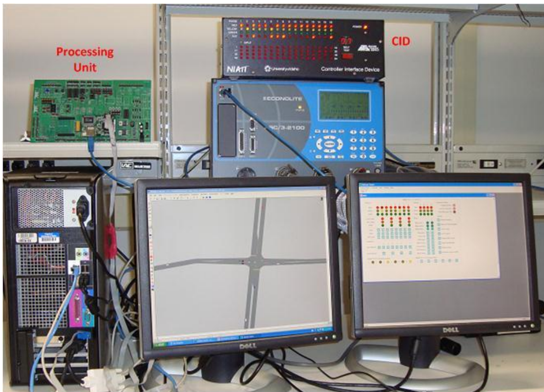
Figure 5. Hardware-in-the-Loop Model Laboratory Setting - University of Idaho's traffic controller laboratory – Moscow, Idaho
