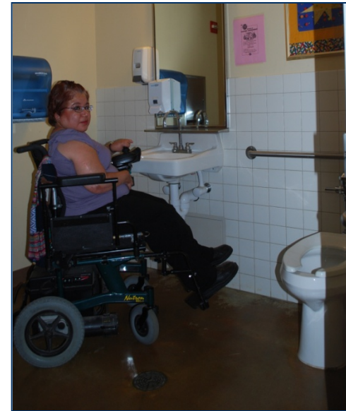
Accessible restroom with cutout sink and grab bars
