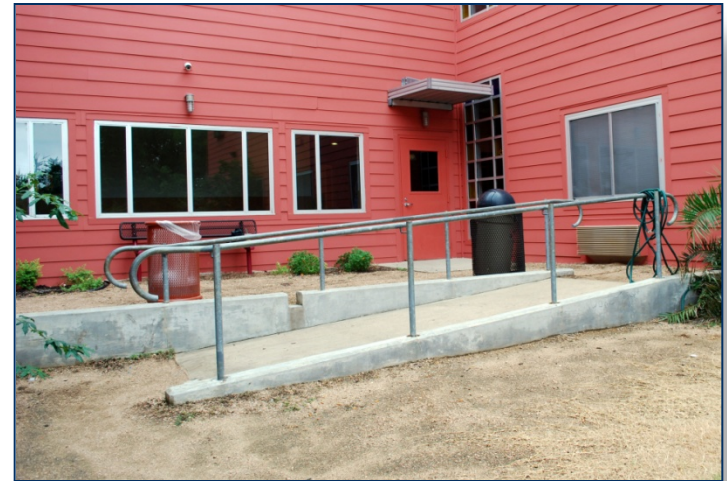
Ramp to emergency shelter patios
