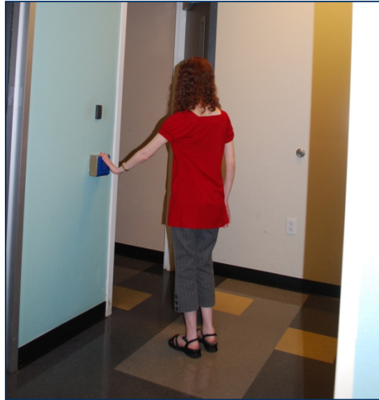
Switch plate entrance to areas where non-residential services are provided
