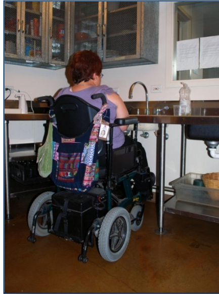
Accessible sink and under counter area
