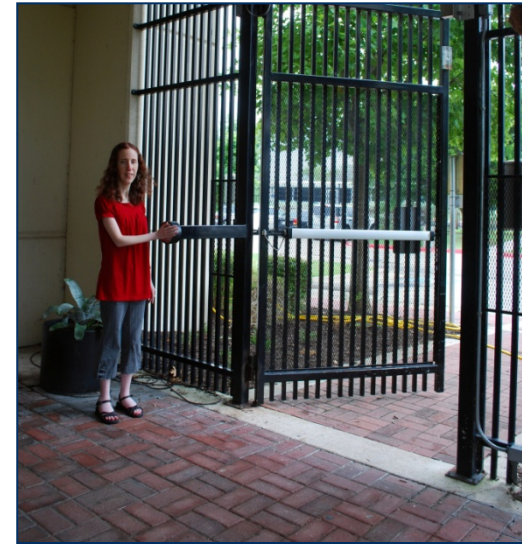
Accessible security gate entrance/exit to building
