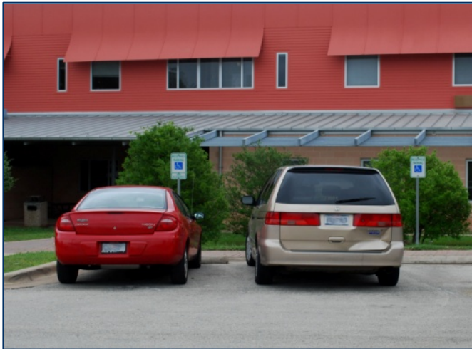
Accessible parking at the emergency shelter
