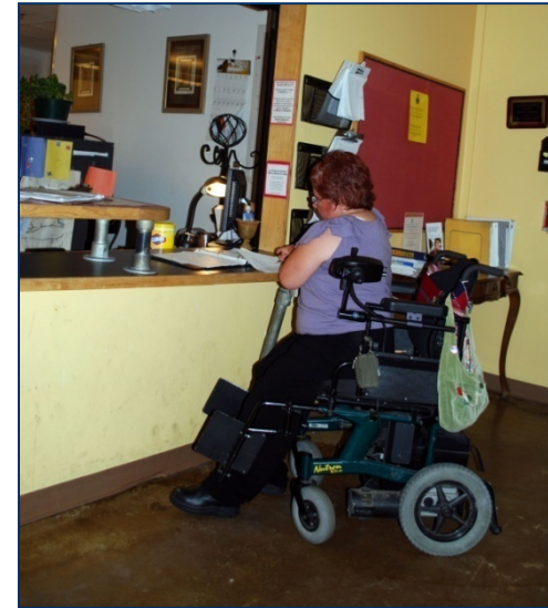
Accessible counter cutout at front desk
