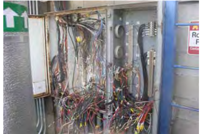
BEFORE – TBX-1 terminal box during initial demolition
