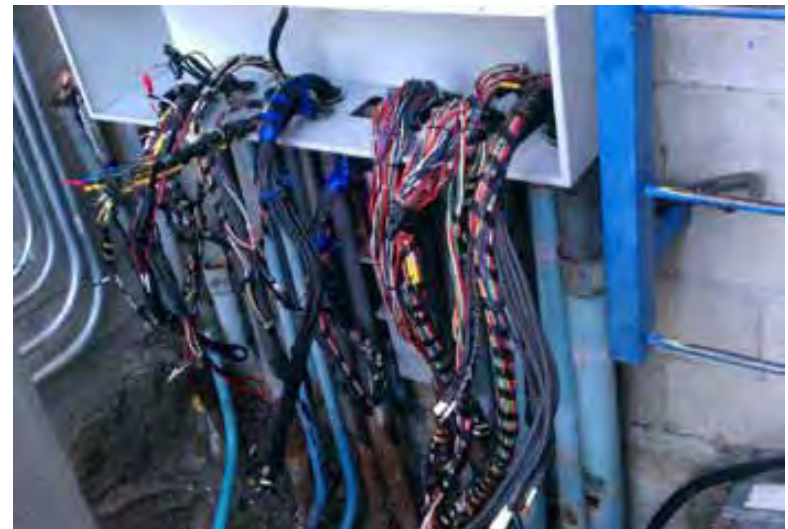
AFTER – Wires neatly grouped just beneath the yet-to-be-installed new terminal box.
