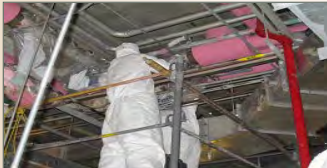
Insulators removing asbestos in duct level
