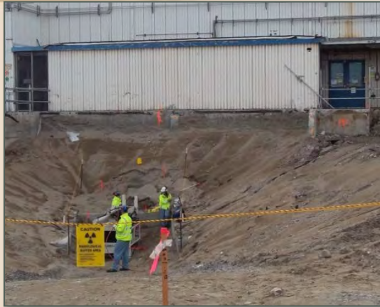
Radiation measurements being taken under the B Cell
