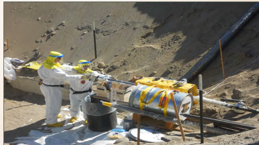
Custom designed tools were remotely operated to remove 12,000 curies of radiation from B-cell
