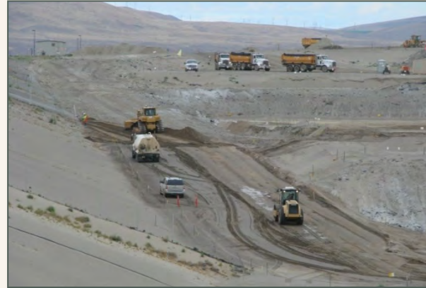
Constructing New Access Ramp into ERDF
