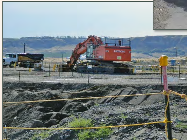
Trench excavation at 618-10 Burial Ground
