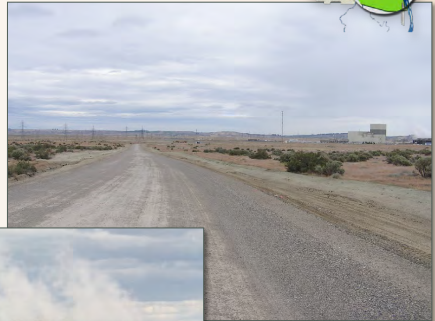
Completed access road for 618-11 infrastructure construction
