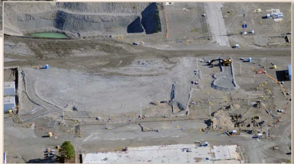
After demolition and backfill
