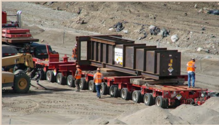
Disposal of 309 Fuel Examination Cell at ERDF
