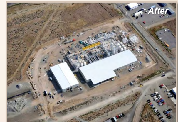
200 West Pump and Treat System
