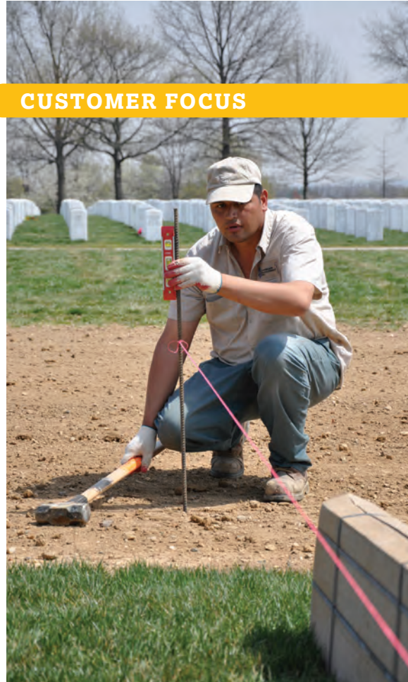
Miguel Canales plumbs a steel rod to assist in aligning headstones at Arlington National Cemetery. Management of contracted services for the nation’s most active cemetery was assumed by Mission and Installation Contracting Command last summer. (U.S. Army Photo by Daniel P. Elkins)
