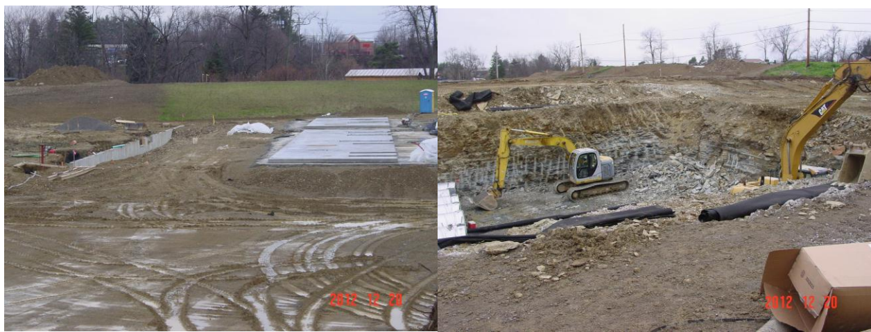
Rear wall on the pouring pad ready to stand-up someday.
