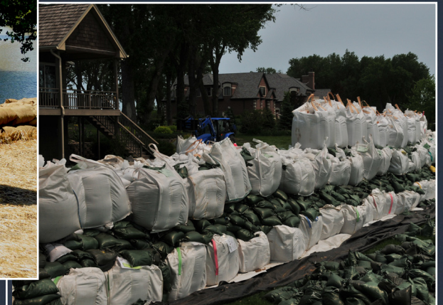
A sand bag barrier was constructed to protect private property from rising Missouri River waters in North Sioux City, South Dakota. The sand bags were put in place primarily by South Dakota Army National Guard Soldiers in anticipation of record flooding along the Missouri River.
