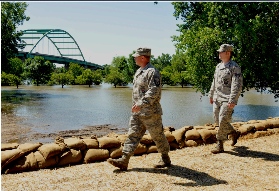
Master Sgt. Clint Thomsen (left) and Staff Sgt. Ryan Baker, with the 185th Air Refueling Wing (ARW), Iowa Air National Guard, Sioux City, Iowa, monitor levees built along the Missouri River near the Siouxland Veterans Memorial Bridge. The two airmen are checking for potential problems along the levee on June 15, 2011.
