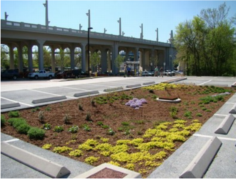
Figure 3: View of Chattanooga, Tennessee's Renaissance Park Rain Garden
