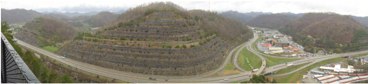
Figure 4-47: The Pikeville Cut-Through. Two ridges were cut through, which allowed the river, a major highway, and the railway to be re-routed. Soil and stone removed from the mountain filled the former riverbed, which was redeveloped as part of Pikeville. Remaining rock and soil filled nearby mountain hollows to create flat land for ball fields and other public facilities.
