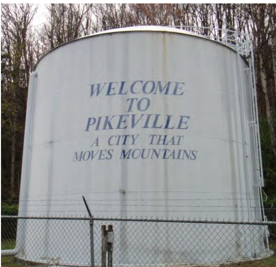
Figure 4-48: Water tank in Pikeville.
