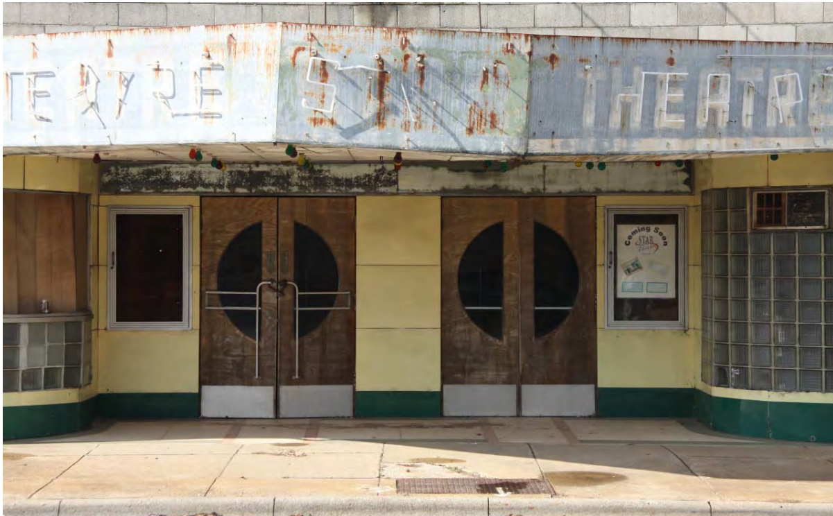
Figure 4-96: The Star Theatre entrance and marquee in downtown Moulton
