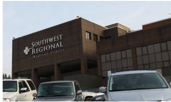
Figure 4-11: Southwest Regional Medical Center was identified as an important asset in the county.
