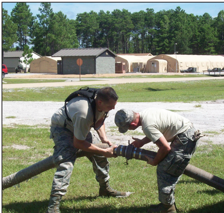
Airman 1st Class Matthew Monk and Staff Sgt. Eugene Renney, both from the 445th Civil Engineer Squadron, connect sections of water lines for the base water distribution system during Silver Flag 2010.
