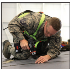
Maintainers work hard during ISO inspection
