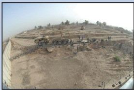
Deployed reservist part of fence build up
