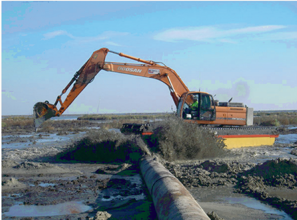
The sediment from the river is delivered from the river to then newly created marshlands.
