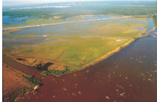
Aerial view looking north depicting the marsh created within the Bayou LaBranche project area. Lake Pontchartrain is in the foreground, U.S. Interstate 10 can be seen running east to west near the top, and the emergent marsh (open water prior to 1994) is the large, vegetated area in the center.
