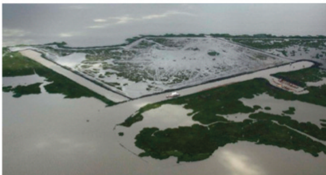
Aerial view of the east end of Marsh Island after commencement of construction activity.
