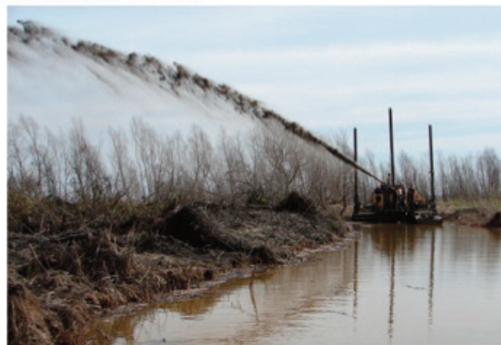
Small spray dredge enlarging the Grand Volle Ditch and spraying the spoil over existing marsh.
