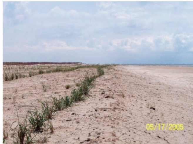
The plants and sand fencing shown above will help to maintain the integrity of Timbalier Island by capturing and retaining wind-blown sand.
