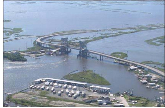
LA 1 Bridge in Leeville, Louisiana
