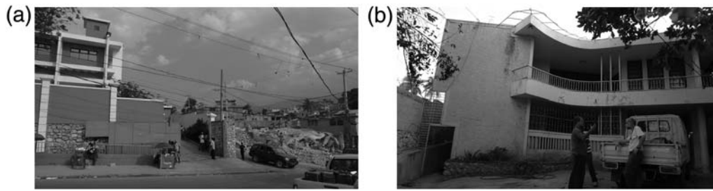
Figure 2. (a) A good-quality commercial structure in which MMI V–VI is estimated based on an eyewitness interview. (b) A private home, masonry C construction for which MMI VI is estimated. The structures on both sides of the structure shown in (a) collapsed catastrophically, as did a school building adjacent to the house shown in (b).
