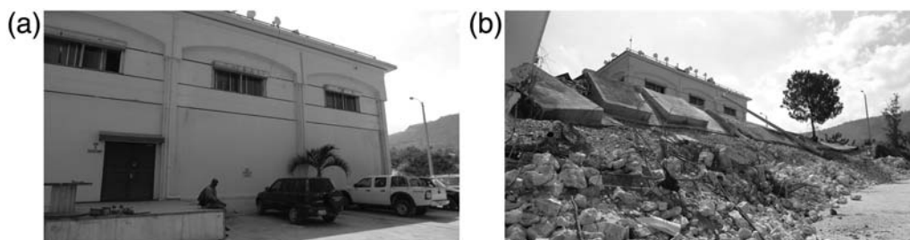
Figure 3. (a) Canape Vert Voila cell phone facility. (b) Collapse of the retaining wall in the parking lot. The face of the building seen in the photograph is aligned roughly north-south; the battery racks discussed in this study are located on the ground floor in a large room behind the doors seen in (a).
