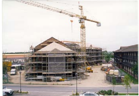
A one-plus-one dormitory under construction in the 1990s
