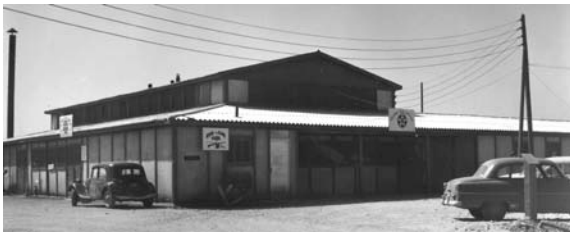
Chaumont Air Base Post Exchange Building, 1955
