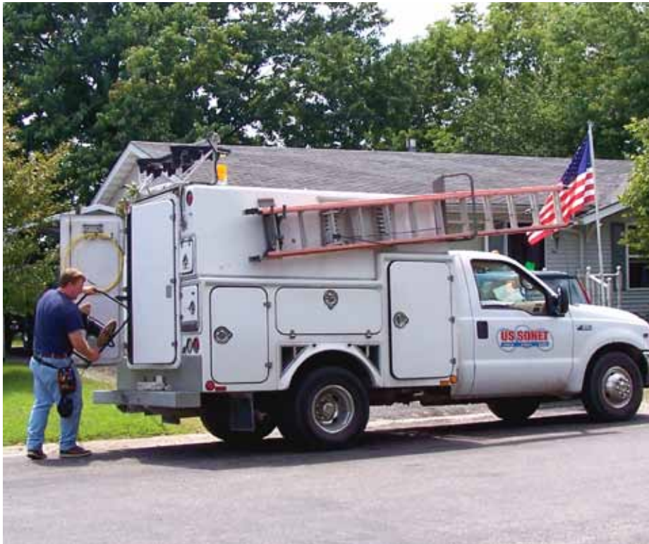
This US Sonet engineer is installing residential cable service in Salem, Ill. US Sonet was able to bring a fiber optic network of underground cables, for Internet, phone, and cable TV services, to rural, south central Illinois through financing from Jefferson Marion Washington CDC.
