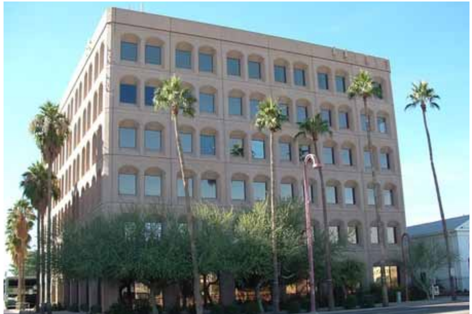
Three Native American human services providers are sharing this building in downtown Phoenix. The building was renovated with gap financing from MultiBank.
