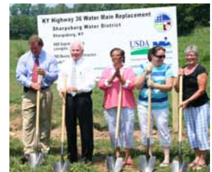
The Sharpsburg Water District breaks ground on a new water line project.
