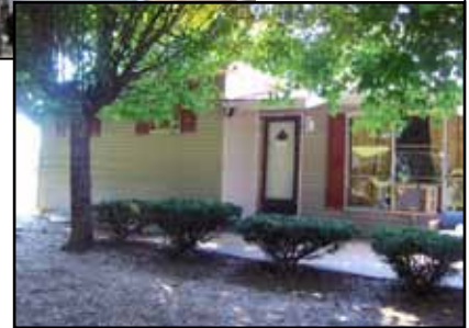
Before and after photos of a home improvement project made possible with RD's home repair program.
