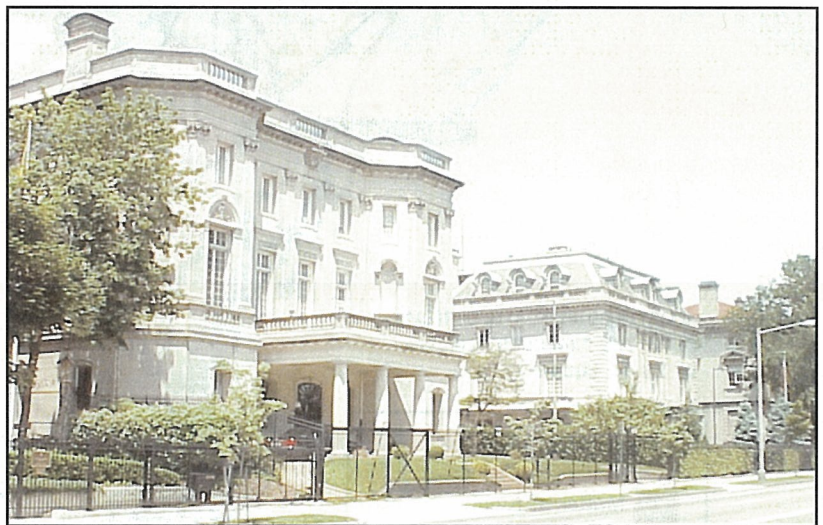
CHANCERIES AND CHANCERY ANNEXES ON 16TH STREET, NW
