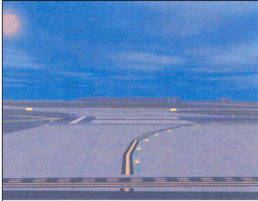
FIG AD 1.1-14 Taxiway Lead-On Light Configuration
