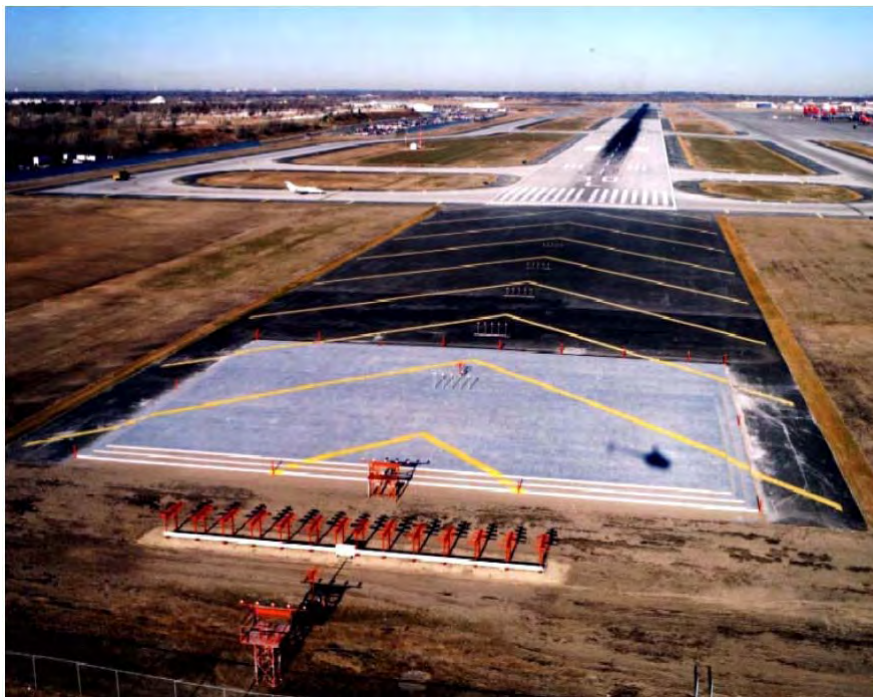
FIG AD 1.1-56 Engineered Materials Arresting System (EMAS)
