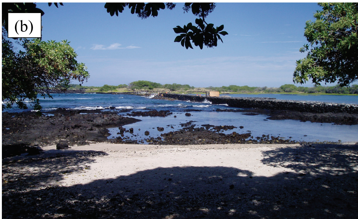
Figure 4. Kaloko fishpond wall during restoration on 11/29/04. (a) View north from pond edge just inland of wall. Structure extending into pond from wall is makaha, or sluice gate. (b) View north from seaward side of wall. Restoration of the southern portion of the wall is complete; masons are visible working on the central portion. Photos by D. Hoover.
