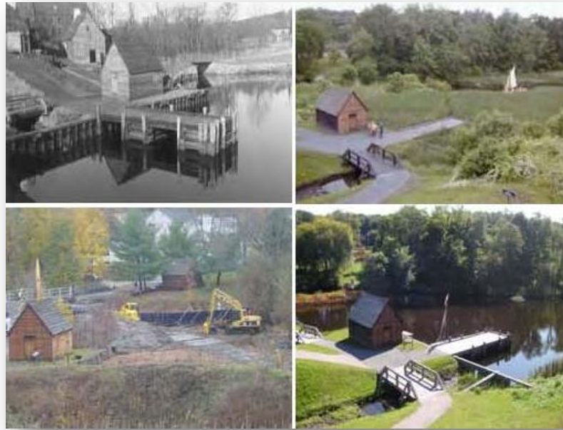
Figure 3. Images of the turning basin over time: circa 1954 (top left), August 2007 (top right), October 2007 (bottom left), and September 2009 (bottom right). (Photos courtesy of NPS 2009a and M. J. James-Pirri.)
