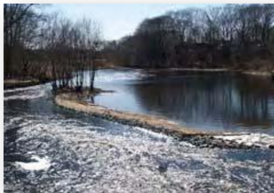
Figure 6. Gravel berm built during restoration to protect stream riffle habitat for rainbow smelt spawning, shown at spring high water, 2009 (photo courtesy of NPS).
