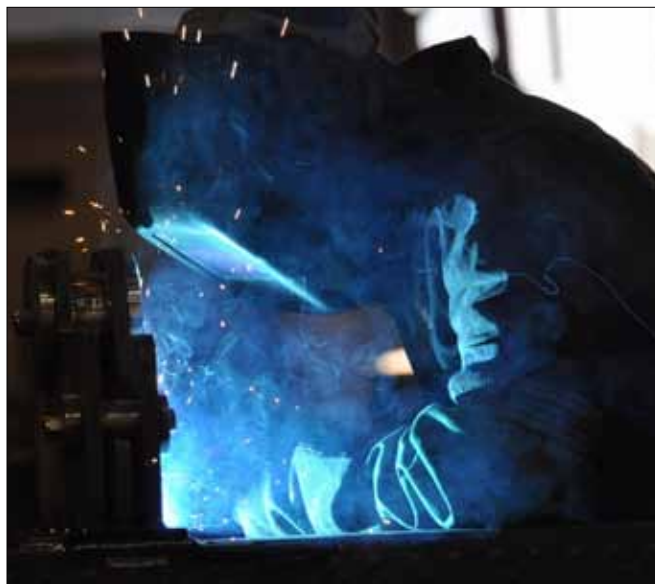
An AECOM-CACI FIRST Allied Trades contractor welds the deck plate onto the Bastogne bumper before installing on an M-ATV.
