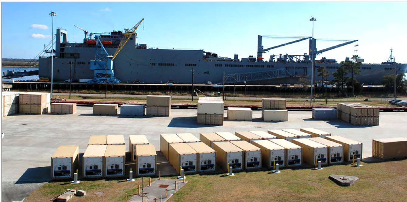
Containerized cargo will soon be driven onto the USNS Red Cloud at Wharf Alpha, Joint Base Charleston. At least 20 acres of land must be available to provide a staging area for loading and unloading a ship like the USNS Red Cloud.
