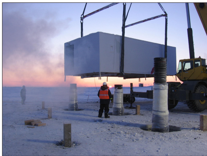
Figure 3. Installation of the Deadhorse, Alaska, observatory, January 2010.
