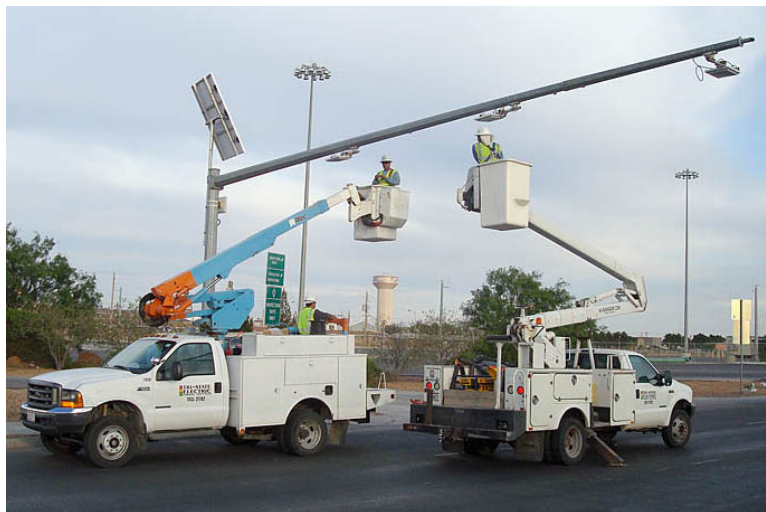
Figure 10. Installing RFID antennae on a mast arm.
