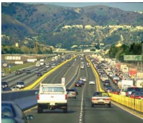
Plastic pylons separate priced lanes from free lanes on State Route 91.
