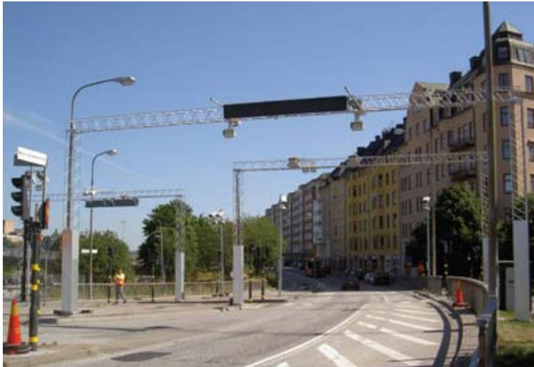
In Stockholm, electronic tag readers and cameras are installed overhead on gantries.
