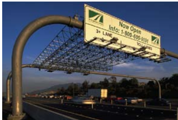
Transponders are read by overhead antennas, allowing tolls to be paid without stopping.
