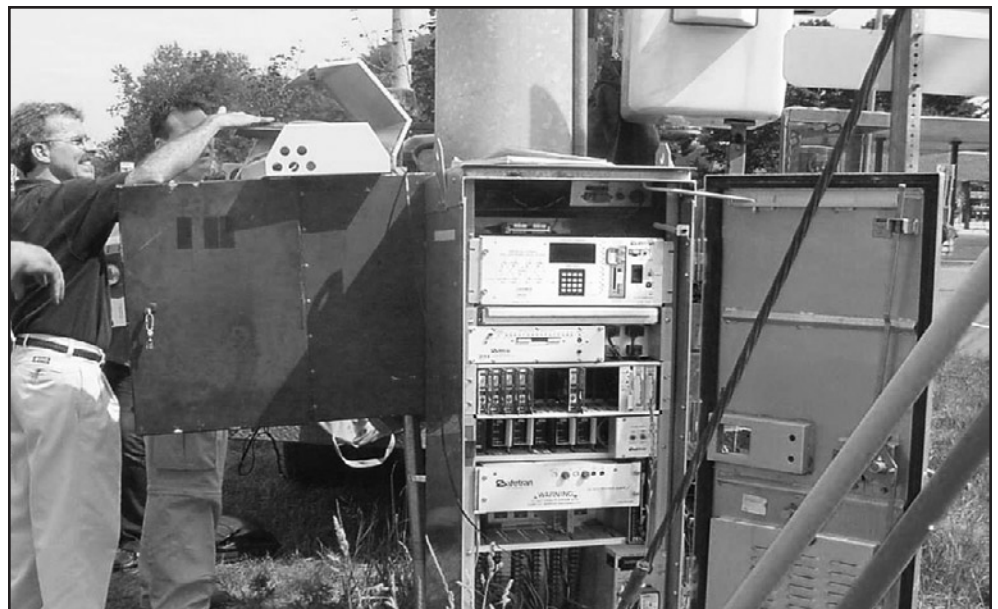
Figure 15. CCTV Camera and Signal Control Software Installation
