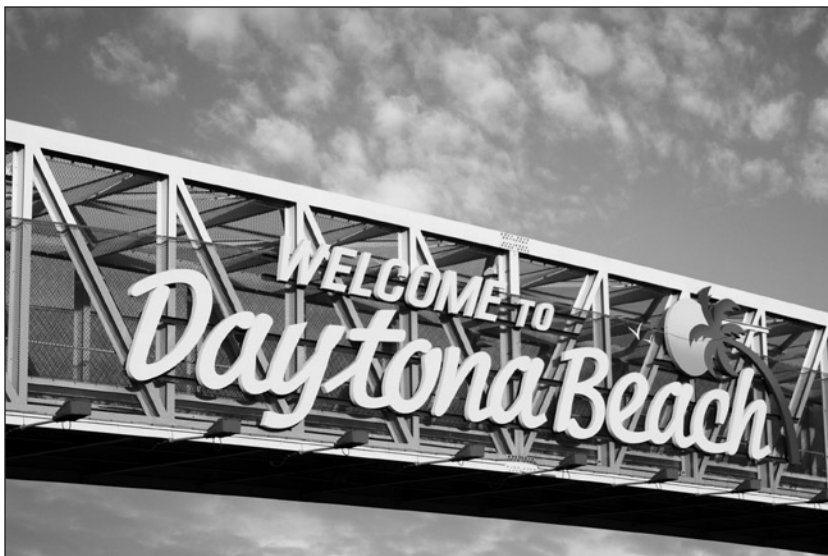
Figure 12. Pedestrian Walkway Leading to the Daytona International Speedway
