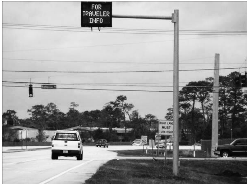
Figure 14. An FDOT Permanent DMS on a State Arterial Directing Event Traffic
