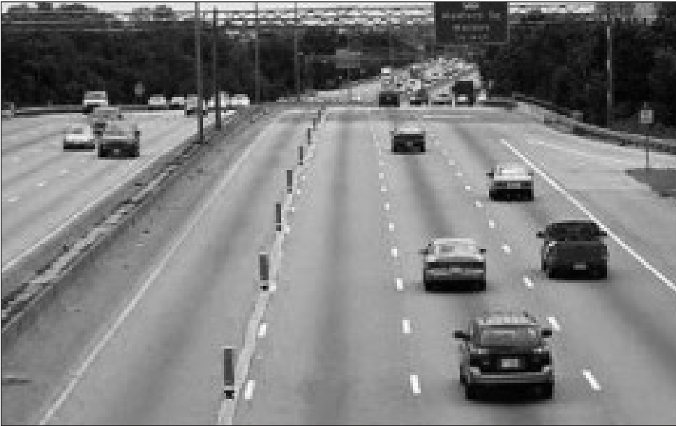
Figure 5. Lane Restrictions on I-93 during the DNC
