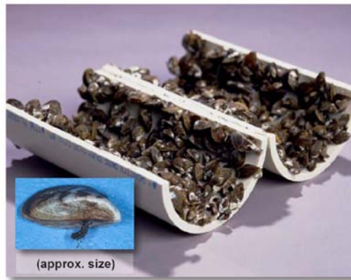
Figure 22: Zebra Mussels Inside a Pipe
