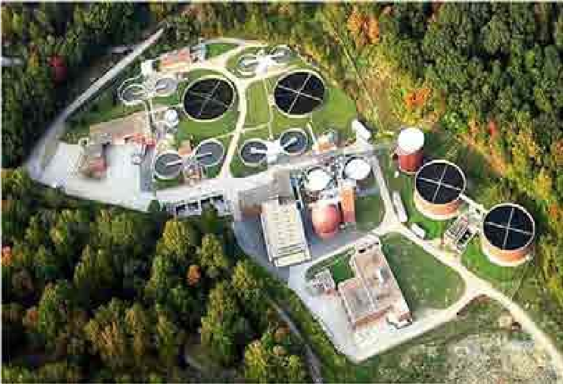
Figure 10: Municipal Wastewater Treatment Facility – Potential Non-Traditional Water Source
