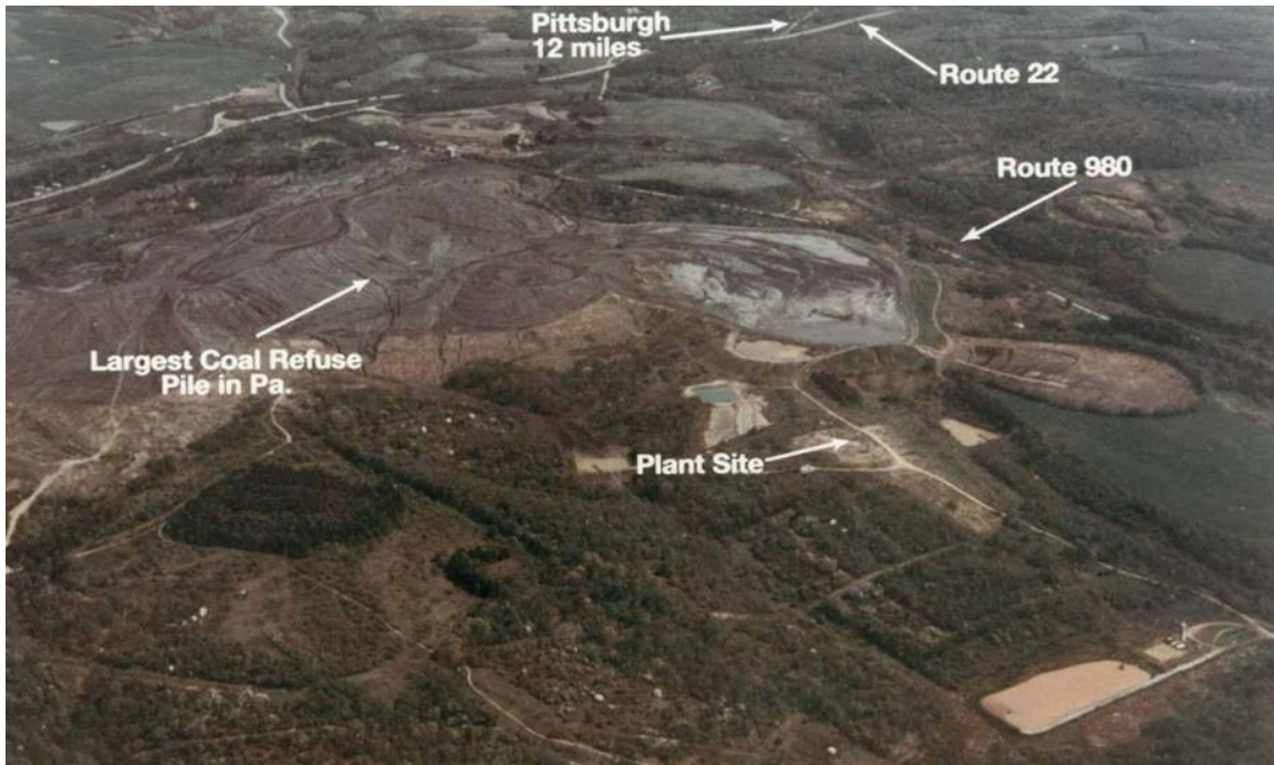
Figure 6: Beech Hollow Power Plant Site
