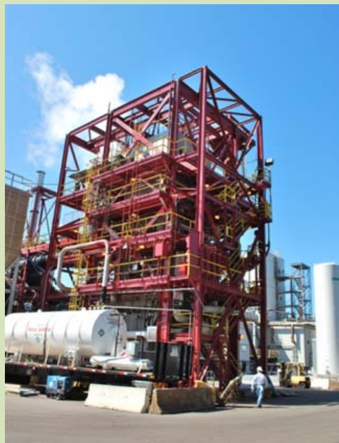
Alstom's 15-MWth Boiler Simulation Facility
