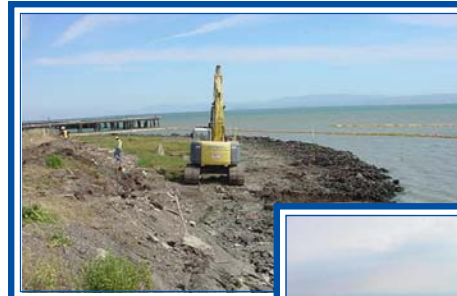
Metal Debris Reef Prior to Excavation (Before)
