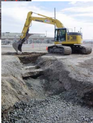
Backfilling Trenches in Parcel B
