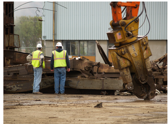
Demolition of Building 408 Furnace
