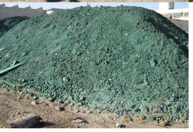
Use of water based soil stabilizer to cover stock piles. Mixture binds with loose soil to develop a exterior crust to the piles. In addition to stockpiles, stabilizer will be applied to trench excavations.
