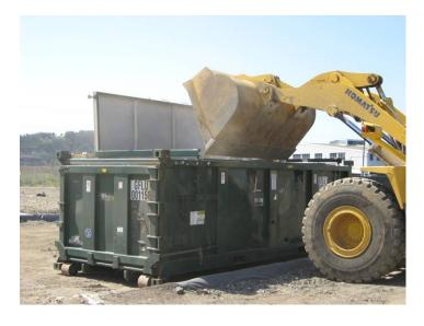
Radiologically impacted soil is loaded directly into bins with locking covers and placed in secure areas prior to off-site disposal
