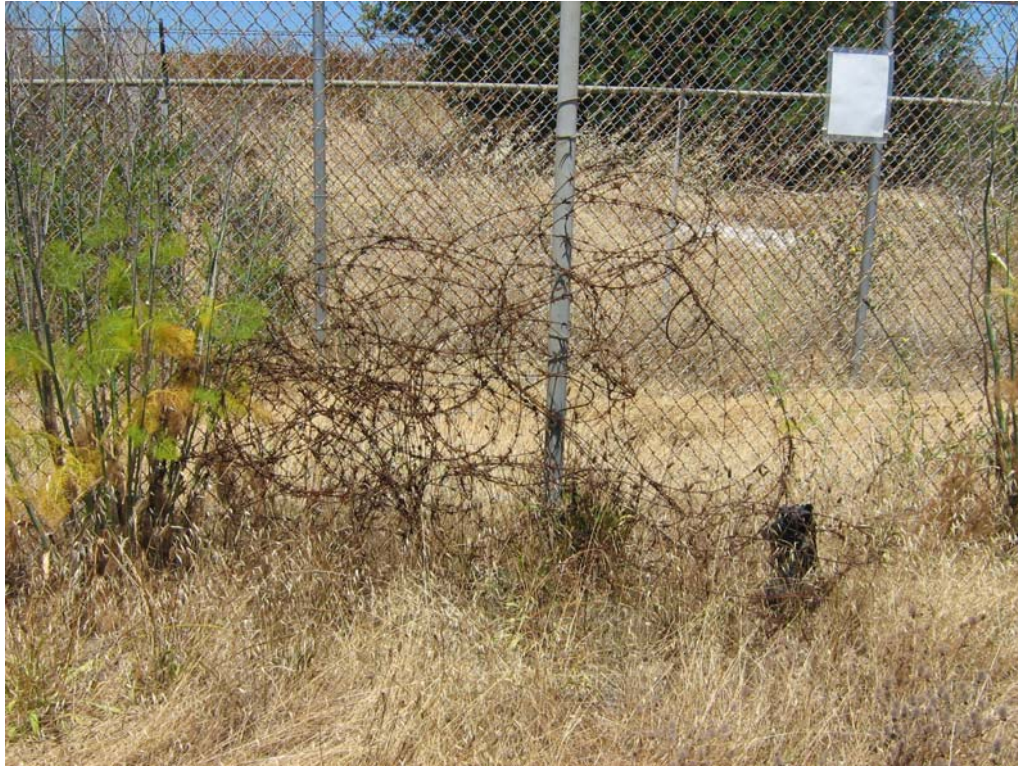
Repaired section of northwest perimeter fence for Parcel E-2.
