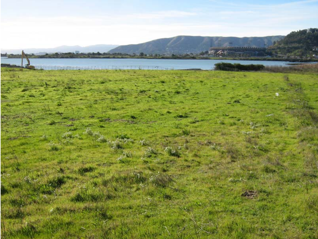
Facing west from landfill cap, December 30, 2010 quarterly inspection.
