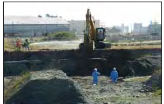
Excavation of soil with lead contamination
