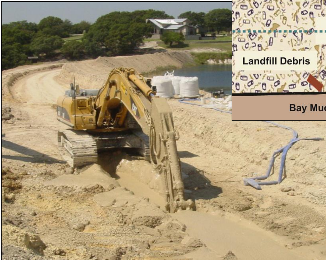
Typical Bentonite Slurry Trench Prior to Backfill with Soil-Bentonite Mixture
