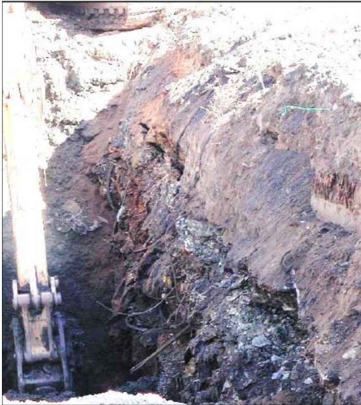
Photo of trench in landfill
