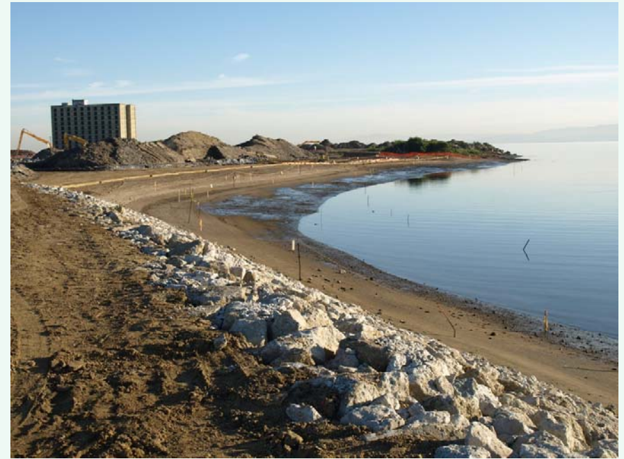
Parcel E-2 shoreline after placing rock (looking south) January 12, 2012
