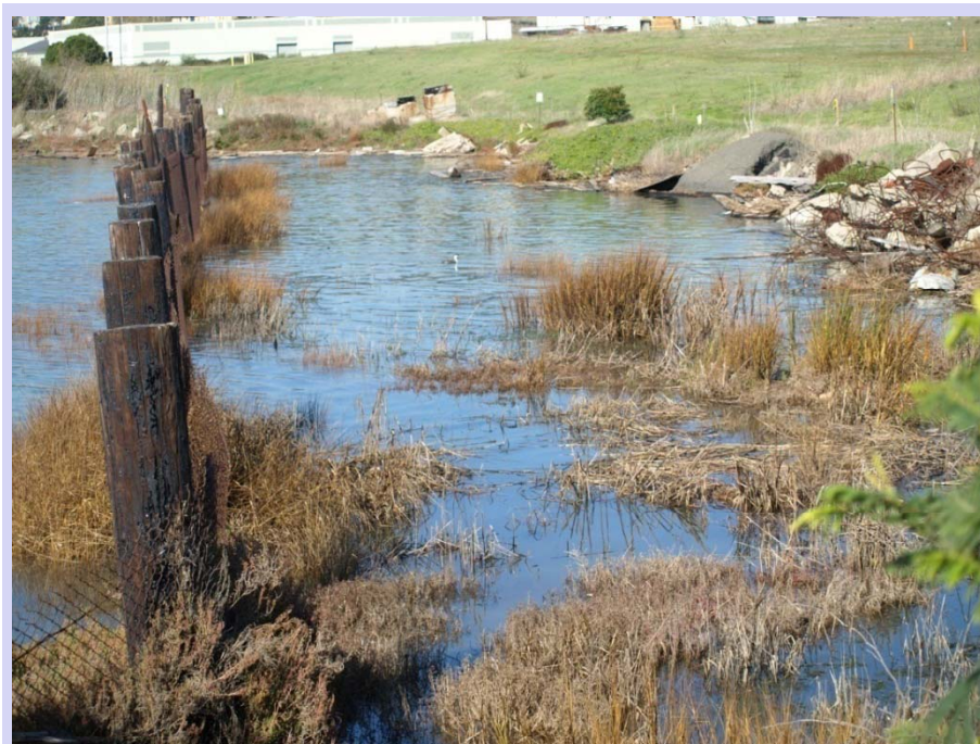
Parcel E-2 shoreline before field work – high tide (looking north) November 17, 2009
