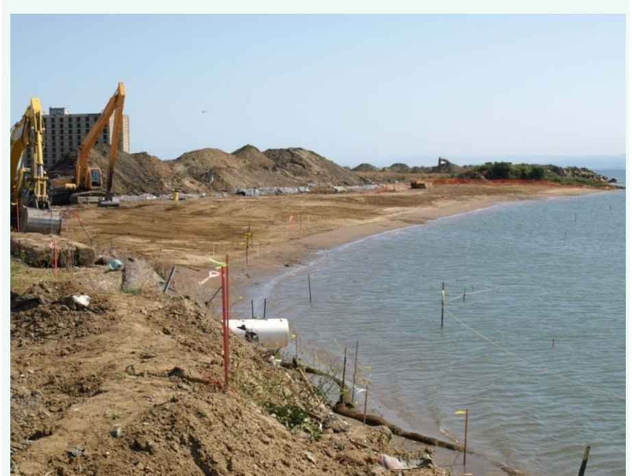
Parcel E-2 shoreline during field work (looking south) September 13, 2011
