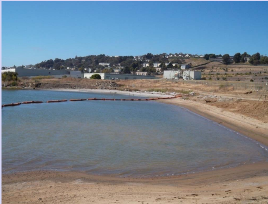
Parcel E-2 shoreline after backfilling (looking north) August 16, 2011
