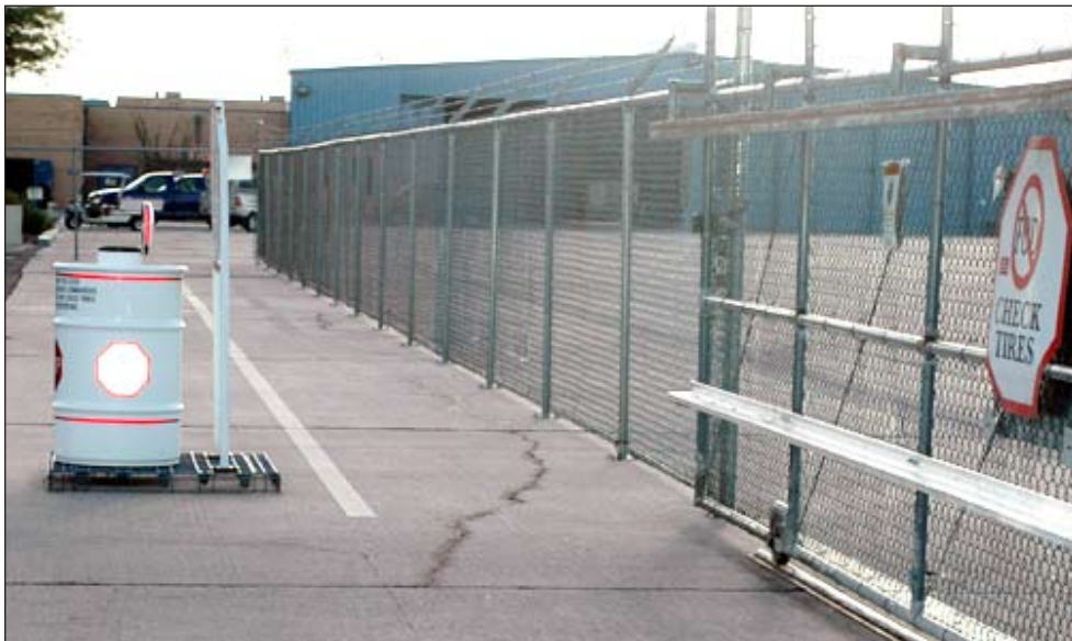
The new south munitions gate and sensor pad were installed and paid for with Repair Enhancement Program funds.
